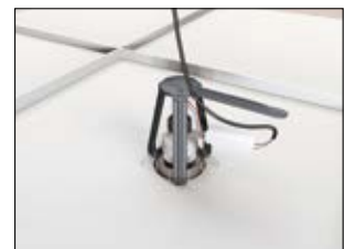
4. Connect the power supply unit and fix the cable in the cable retainer.
