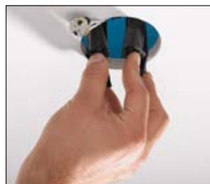
2. Place SpotClip in the desired position.
