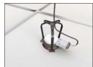
4. Connect the downlight to the power supply and fix the cable into the routing eyelet.
