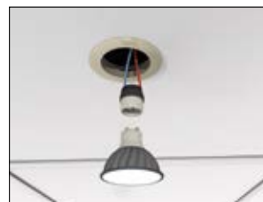
3. Connect the bulb to the socket and lock into the correct position.
