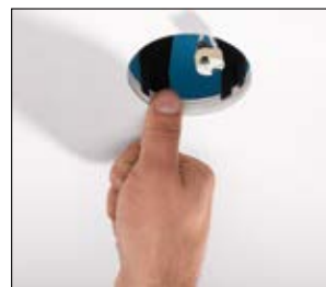
3. Push the spikes into the plasterboard to prevent shifting.
