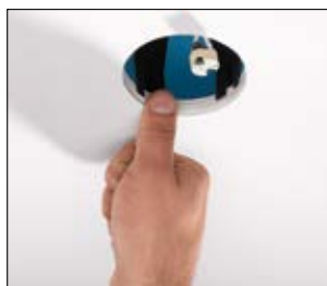
2. Push the spikes into the plasterboard to prevent shifting.
