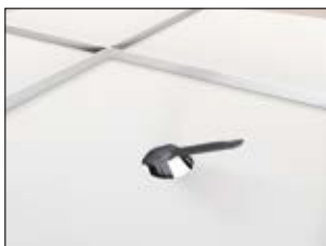
1. Insert the mounting support through the fixing hole.
